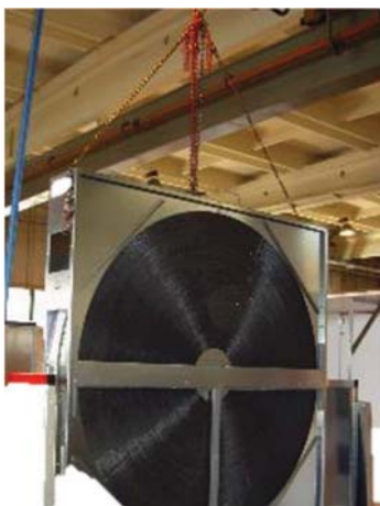
Figure 144: Lifting with chain hoist
