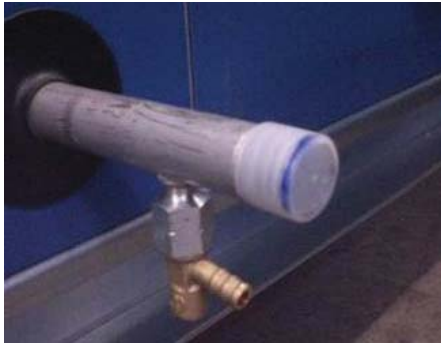
Figure 100: Drain valve
