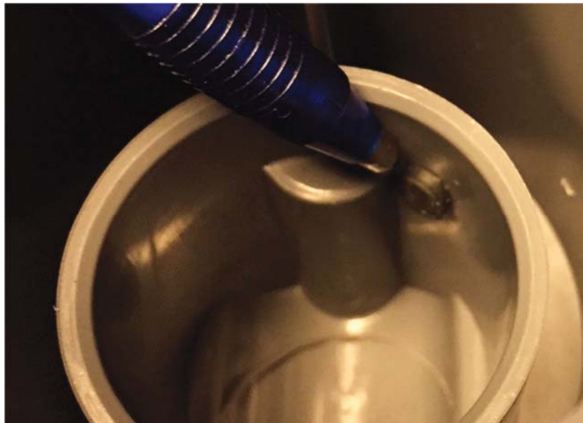
Figure 110: Pressure side installation: remove the black closing plug
