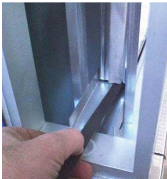
Figure 55: Pulling out the filters
