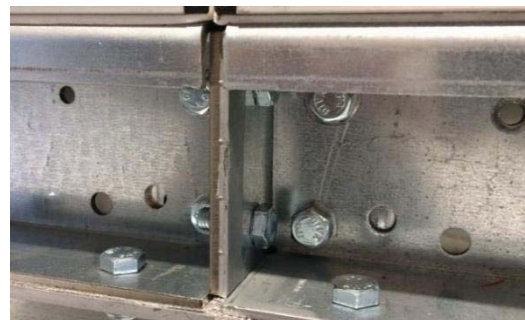
Figure 29: Screw connection of base frames
