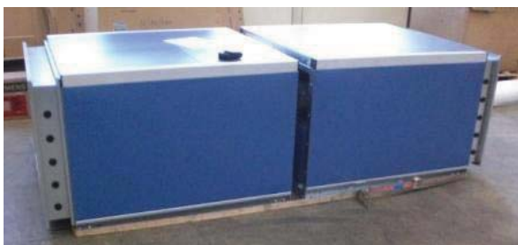
Figure 20: Pulling AHU sections together
