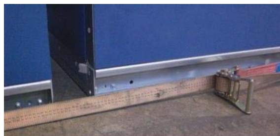
Figure 21: Pulling AHU sections together (detail)
