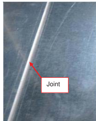
Figure 42: Sealing the section connection (joint) with the sealing agent
