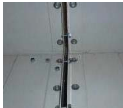
Figure 32: Connection via connection angle
