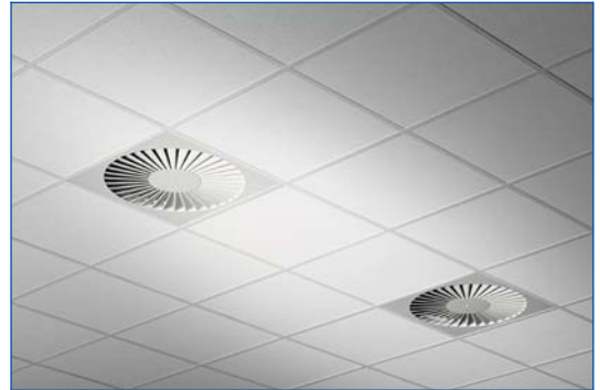
Installation in T-bar ceilings, arrangement in a row
